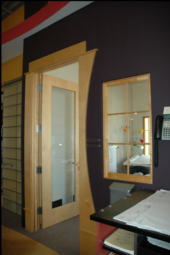
Scraps of wood were used to trim doorways.
